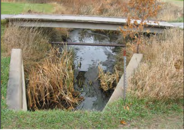
Outfall 005 to Unnamed Creek
