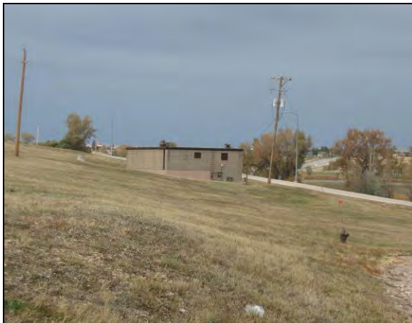
Building 3015 – O/W Separator
