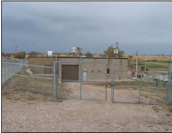
Building 3013 – Pretreatment Facility
