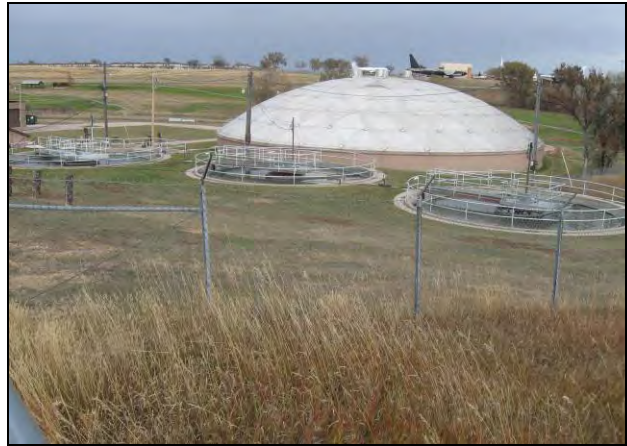
Building 3010 – Trickling Filter
