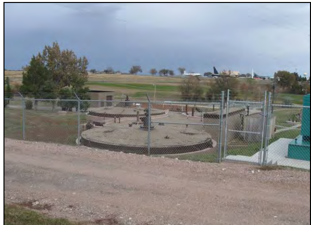
WWTP Facilities Adjacent to Building 3007
