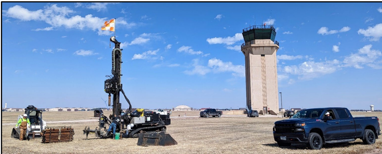
Drilling a new monitor well in 2023
